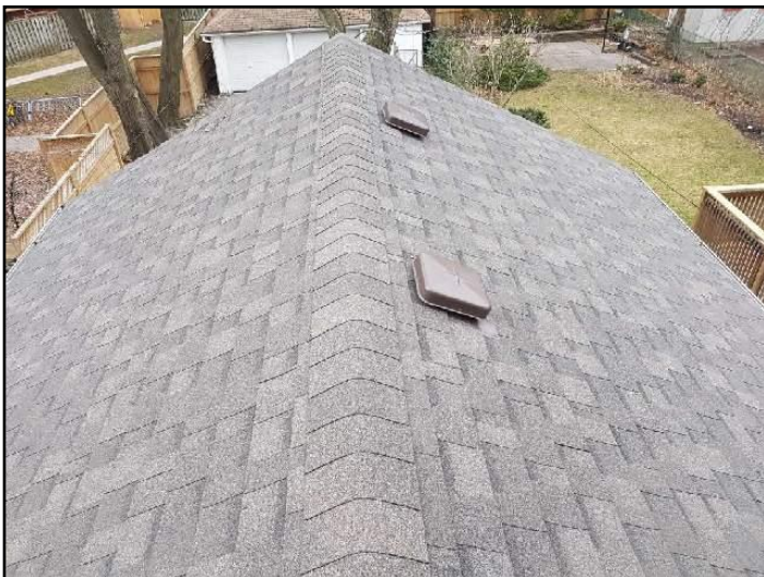
1. Asphalt shingles
