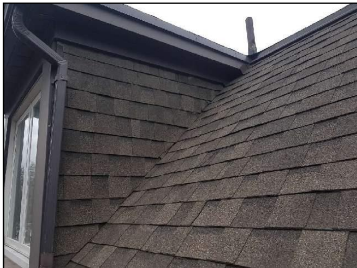
2. Asphalt shingles
