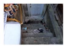
Step(s): rear: requires maintenance, provide handrail
