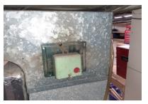
Registers: unusual location for some return units- improve if renovating insulation around some registers may contain asbestos encapsulating the insulation is often the best approach Environmental Consultants can assist if this is a concern
