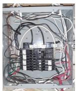
BRANCH WIRING: based on random sampling it was determined the wiring has been upgraded
