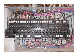
BRANCH WIRING: random sampling determined the wiring has been upgraded throughout
