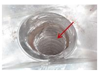
Registers: insulation around some registers may contain asbestos encapsulating the insulation is often the best approach Environmental Consultants can assist if this is a concern
