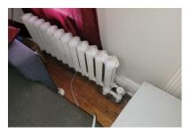
Piping: insulation on heating pipes may contain asbestos encapsulating the insulation is often the best approach Environmental Consultants can assist if this is a concern
