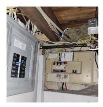
BRANCH WIRING: random sampling determined the wiring has been upgraded throughout
