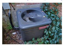
DUCTLESS HEAT PUMP: service annually, repair/replace insulation on refrigerant lines recommend obtaining replacement parts/servicing contract unit provides cooling and supplemental heating
