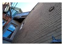
DECK upper deck: older, continue to monitor and repair, some floor boards at exit require replacement, extend railings at sloped roof for safety
