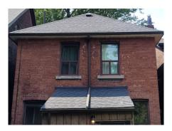
Porch(s): upper porch -asphalt shingles used for flat roof - more prone to leaking - monitor
