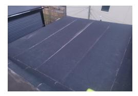
Sloped Surface: overall in good repair, some patched spots- monitor, seal nail heads along edge front dormers (some slate shingles) overall in good repair
