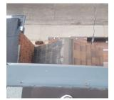
Flashings: chimney/stack: missing proper flashing components, patched instead, monitor Roof/Wall: front: should be sealed properly along northwest wall
